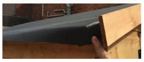
Step 10: Apply the spray adhesive around the edges of the shed and the underside of the membrane. Leave to dry.
