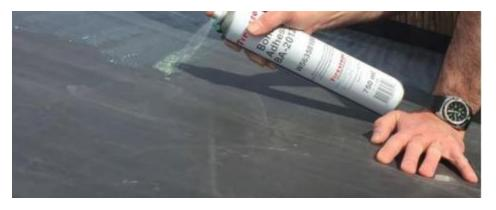
Allow to dry. Use your finger to do a touch test before moving onto the next step
