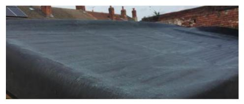
Step 6: Roll the membrane slowly and evenly back over the adhesive-covered exposed half of the roof in stages. Try to minimise air pockets and creasing as you go.
