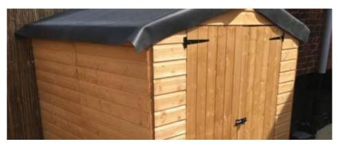
Step 3: Fold half the membrane back on itself and expose the first half of the shed roof working area.
