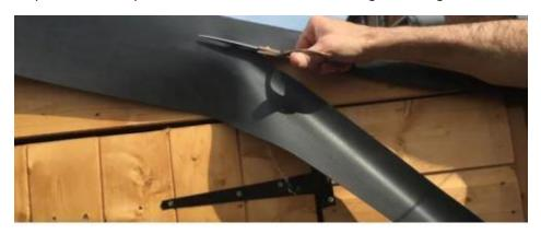
Step 9: At the front of the shed, pinch the corner of the EPDM and fold inwards to form a triangle. Secure with a timber batten strip (not included).
