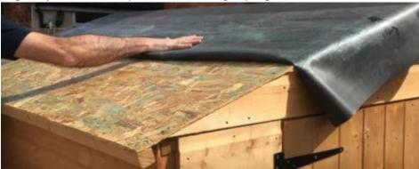
Step 7: Use a soft broom over surface of membrane to ensure full adhesion and to ease out any creases or bubbles.
