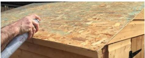
Step 5: Next apply an even coat of spray adhesive to the back of the membrane you folded back earlier.
