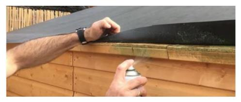
Step 11: Once dry, press the EPDM membrane down firmly by hand, folding the edges.
