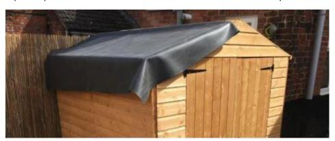
Step 8: Trim off any excess rubber sheet around the edges, leaving a minimum of 50mm overhang.
