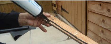
Step 13: Sandwich the membrane overhang between the shed and batten. Fix through the membrane into the shed. Ensure the fixing is below the sealant bead for a watertight seal.
