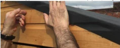
Step 12: Take your timber battens (not included) and run a bead of sealant (included) along the full length of the underside.
